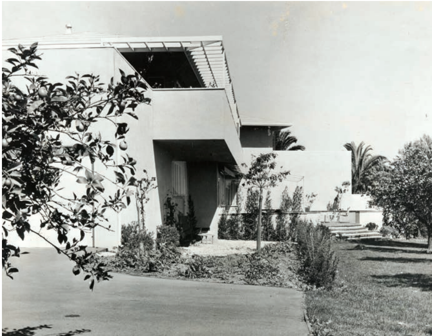
Above: Historical views of the Thomas Mann House
